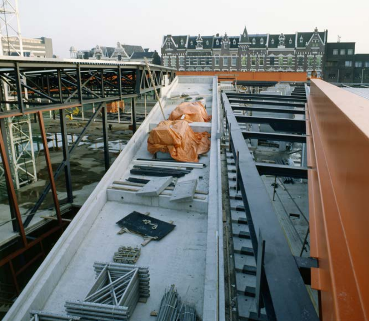
P 8.9 Skew Ramp. Left: Vierendeel truss along Hall 2, after the bend reinforced by diagonal bracings.
